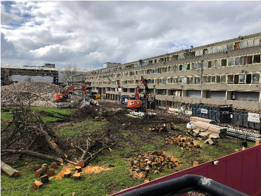
Figure 4. Demolition of the blocks behind Chiltern House (Photo: Loretta Lees, 2018).
