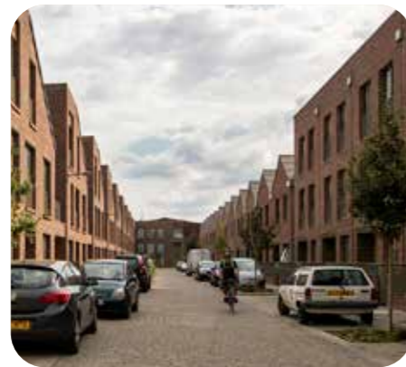
Street parking, and accessible parking for residents along the new lane.
